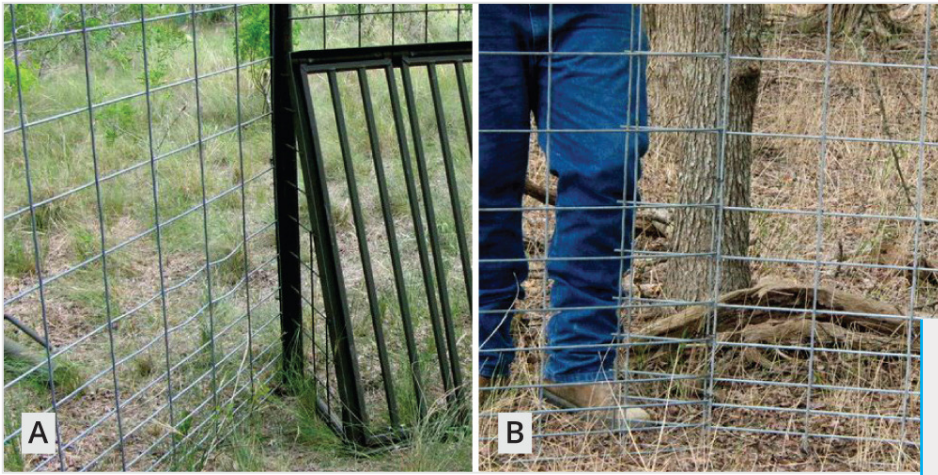
Figure 5. A panel secured to a head gate T-post with doubled wire (A). The remaining panels are attached to one another. It is important to overlap the ends of the panels (B).
